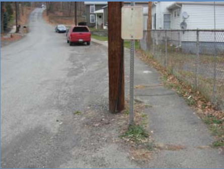
Faded No Parking sign on Exchange Street is not of breakaway design
